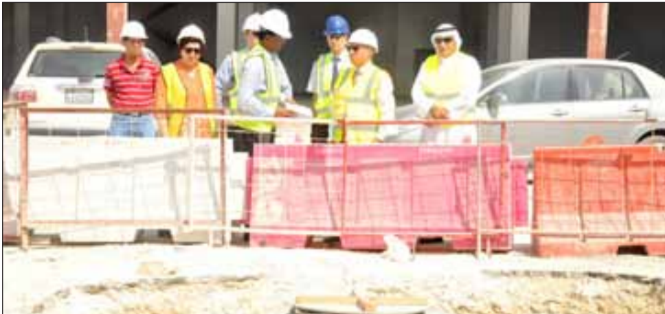
■ Works Minister Essam Khalaf inspected East Riffa sanitation project and gave directions to speed up the work by increasing field visits and the workforce. He was accompanied by sanitary engineering assistant under-secretary Khalifa Al Mansoor and the sanitary projects and planning director Asma'a Murad. They were informed that 40 per cent of the project was completed.
