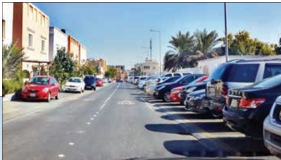
■ Work included construction of 830 parking spaces
