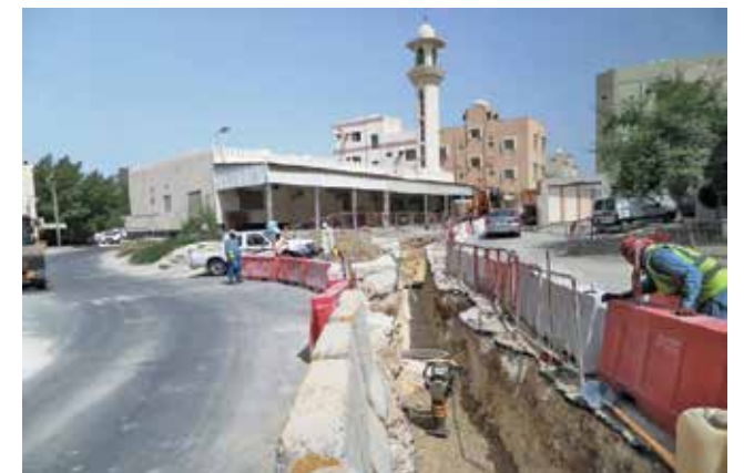
The construction works in progress
